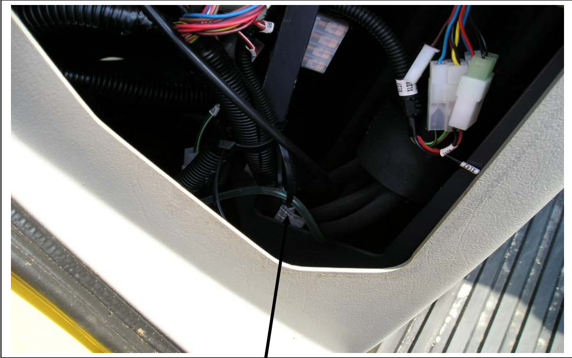
Run hoses and wiring out with the hydraulic hoses.
